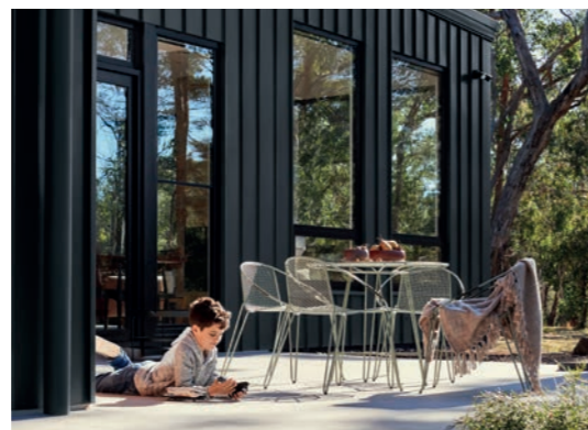
• Walling | COLORBOND® steel Monument® in a Matt finish.
